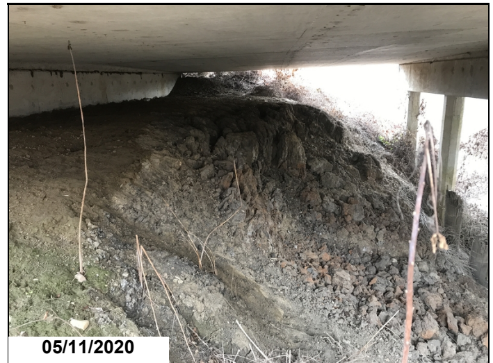
Abutment #2 slope erosion.
