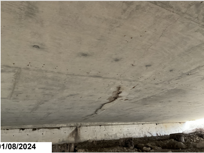
Span #1 soffit-under surface delaminated area and spall.
