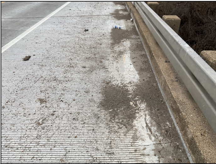
Typical debris in gutters
