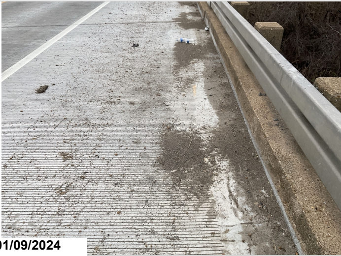
Typical debris in gutters
