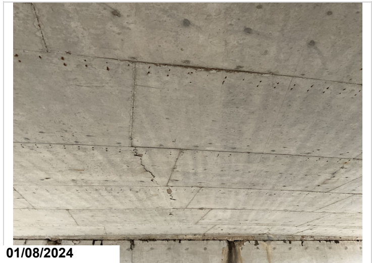
Span #2 soffit-under surface delaminated area.
