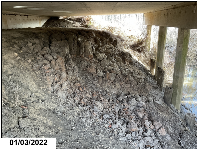
Abutment #2 slope erosion
