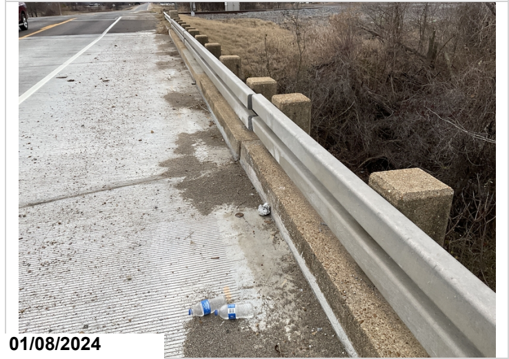
Misalignment from span #2 to span #3.
